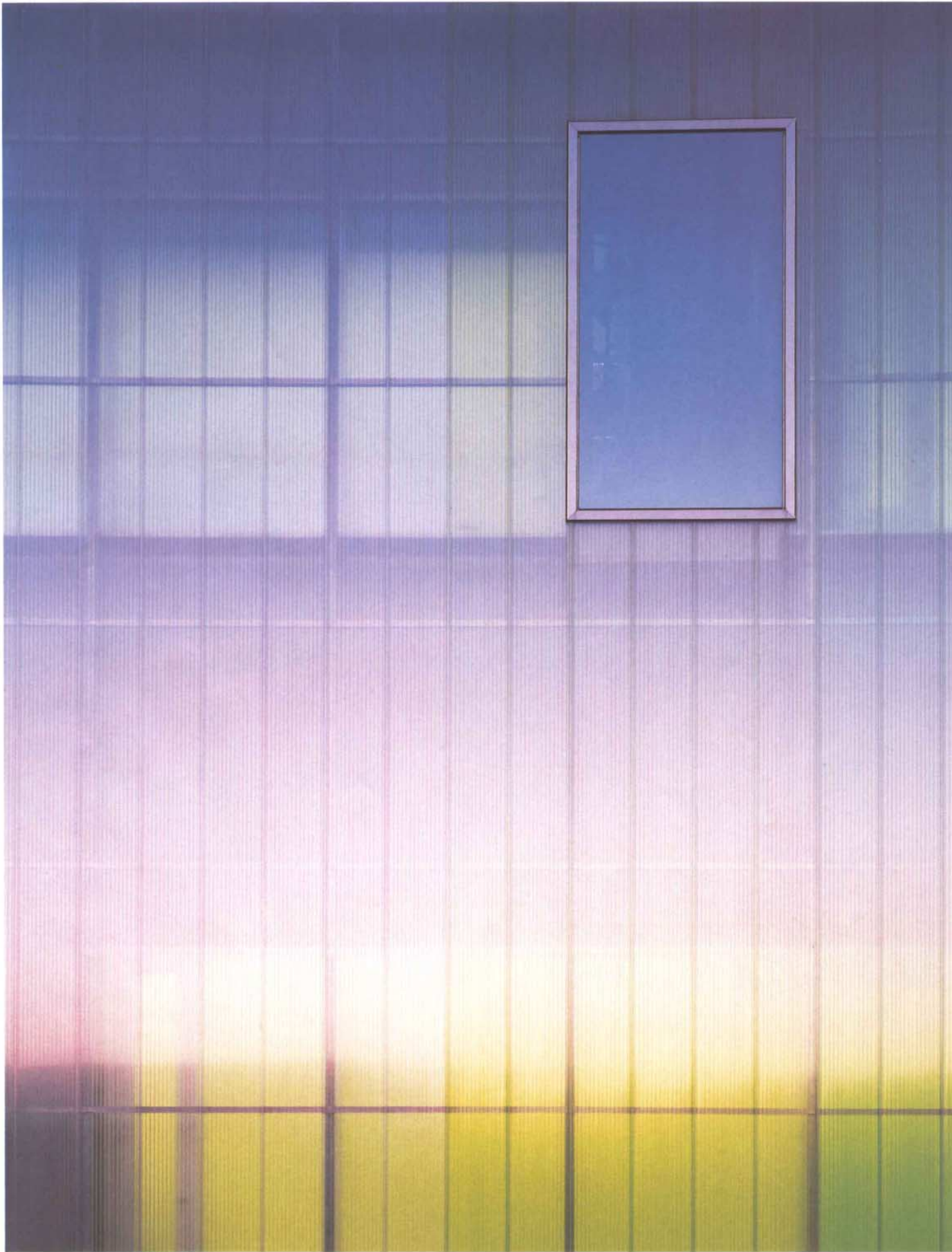
The translucent facade incorporates clear glass windows, so that each studio has a view out.
